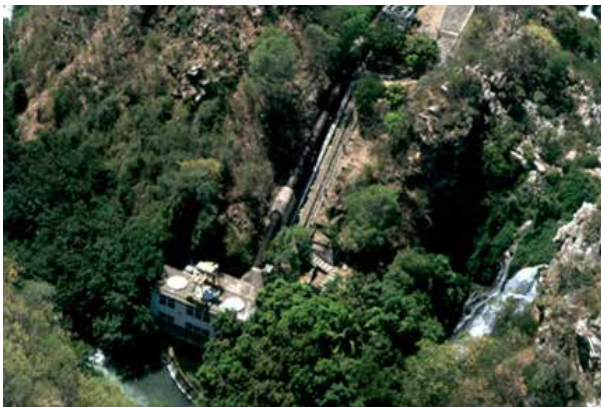
Figura 13: Usina Piloto (CHESF).
